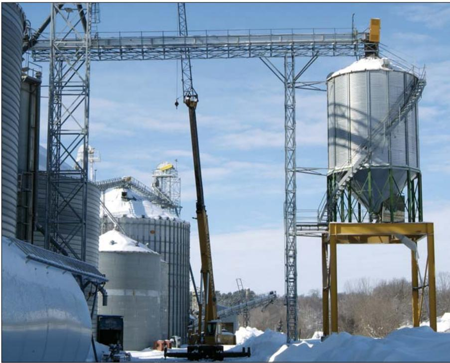
*Rail loadout at Rock Springs runs through an overhead surge bin, served by a new 20,000-bph GSI overhead drag conveyor.*
