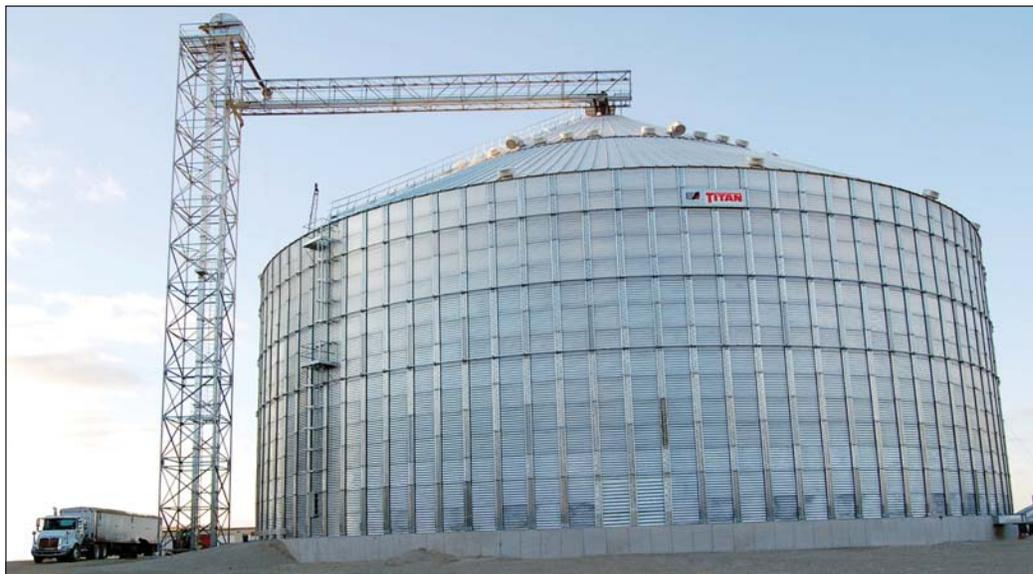
*Above, new ChiefTitan 1.1-million-bushel tank, with its own receiving pit and leg, installed in 2007 at United Cooperative's South Beaver Dam elevator in Wisconsin. At right, a view of the entire elevator. Photo above courtesy of United Cooperative; all other photos by Ed Zdrojewski.*
