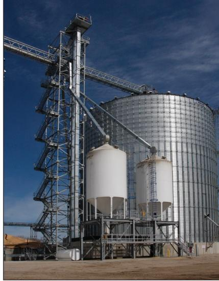
*Ground view showing 15,000-bph Schlagel receiving leg in a 16-foot-x-16-foot LeMar tower, six-hole Schlagel rotary distributor, and two 4,000-bushel Meridian surge tanks.*
