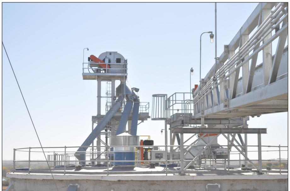
*Rooftop equipment, above, includes the head section of a Schlagel 20,000-bph receiving leg and four-hole Schlagel distributor, as well as a 20,000-bph Schlagel drag fill conveyor. At left, a new 1,000-bushel enclosed receiving pit feeds grain into the receiving leg.*
