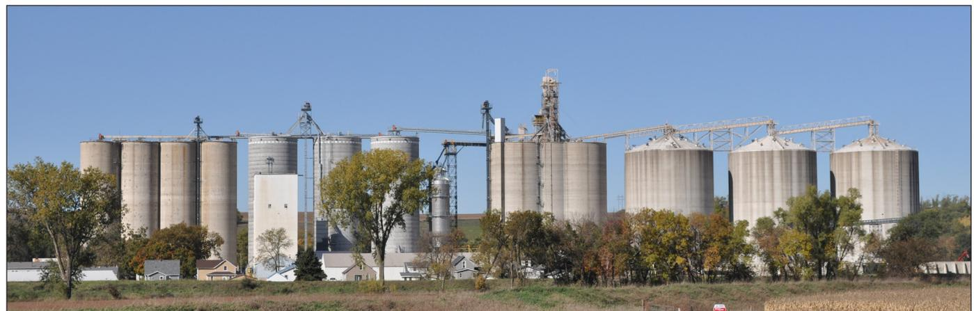
Each tank is equipped with two 40-hp AIRLANCO centrifugal fans plus a 5-hp roof exhauster for aeration at 1/11 cfm per bushel on coarse grains. Two of the tanks have additional 30-hp fans and one a 50-hp fan for air-assist unloading.
