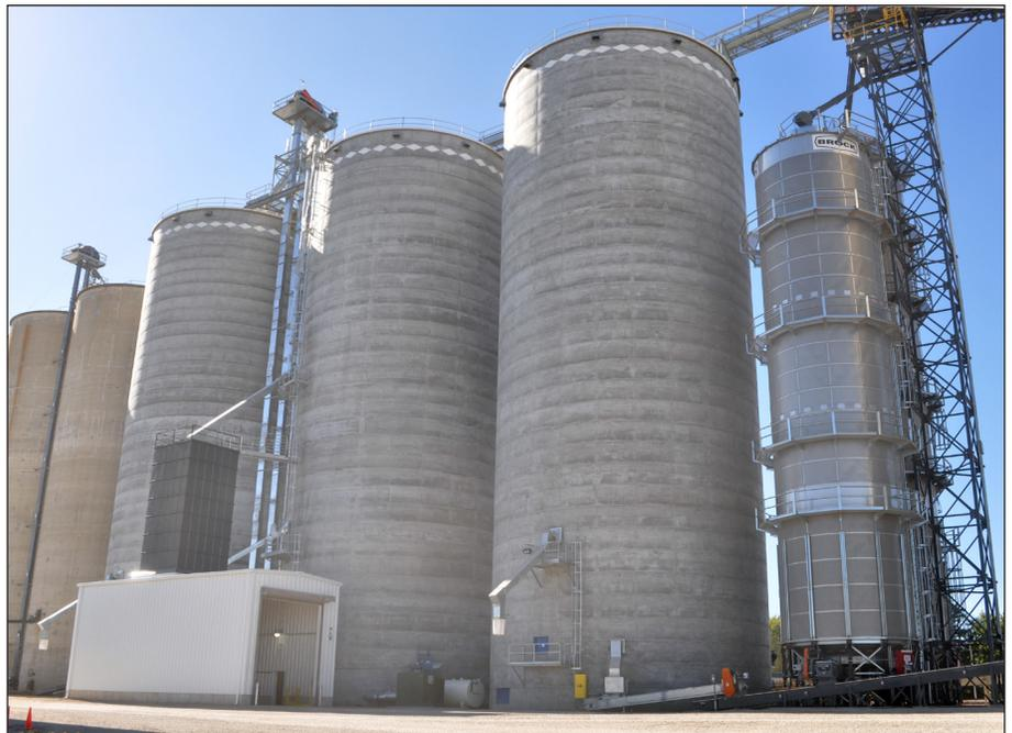
*Closeup view of three new McPherson jumpform concrete tanks, receiving pit, and Schlagel leg, and a Brock tower dryer (not pictured is a Brock 4,000-bph dryer). Ground-level photos by Ed Zdrojewski.*
