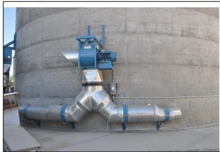
Central Valley Ag's rail terminal at Hinton, IA, below, with three new McPherson jumpform concrete tanks and a Schlagel receiving leg visible just left of center. above, an AIRLANCO centrifugal fan provides power for a KanalSystem aeration and air-assist unloading floor.
