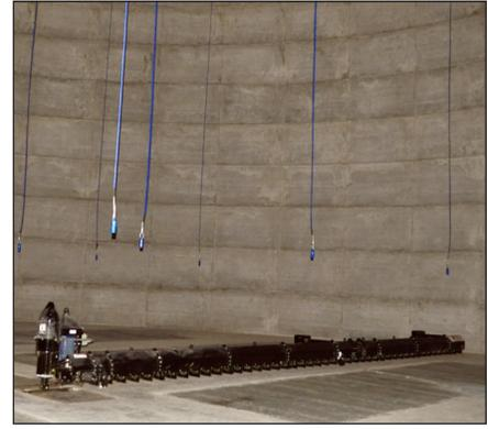
*Daay paddle sweep and TSGC grain temperature monitoring cables inside one of the two larger upright storage tanks.*
