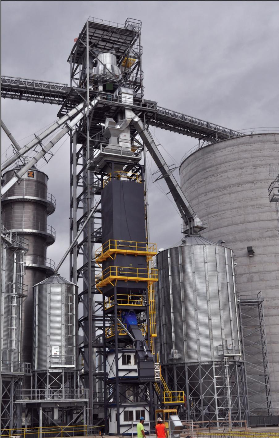
*Grain handling equipment from left includes a Zimmerman 4,750-bph tower dryer, Chief screenings tanks, two Schlagel 30,000-bph receiving legs enclosed in an Allstate support tower, Schlagel rotary double distributor, InterSystems gravity screener, and 60,000-bph CompuWeigh bulk weigh loadout scale.*
