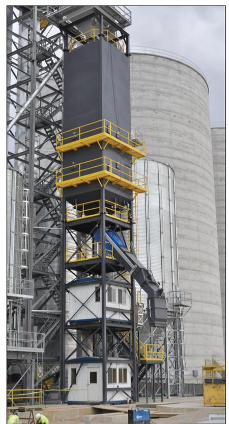
*Closeup of 60,000-bph CompuWeigh bulkweigher for loading 110-car shuttle trains, with Gamet sampler immediately below. Ground level shed is used for official grain inspection.*
