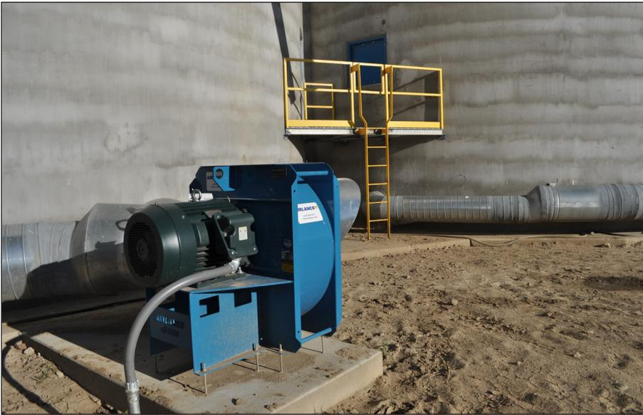
*One 60-hp AIRLANCO centrifugal fan per tank powers AIRAUGER floors for aeration and air-assisted unloading.*
