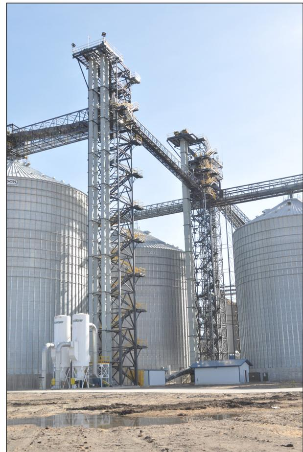
*New 20,000-bph GSI receiving leg (left) enclosed in a Warrior tower outfitted with switchback stairs.*
