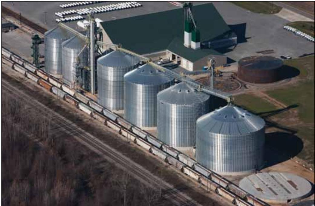
*Sunrise Cooperative Inc.'s 3.7-million-bushel rail terminal near Crestline, OH, with a new 1-million-bushel Behlen tank at far right and the concrete foundation for one of two more million-bushel tanks under construction to the right of that. Aerial photo by Focal Plane Photography, South Euclid, OH.*
