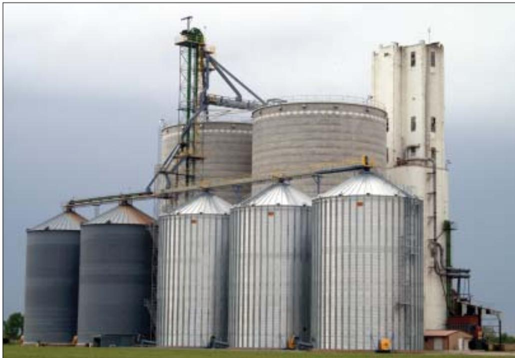
*The Scoular Company terminal elevator at Wellington, KS, with two new 400,000-bushel McPherson jumpform concrete tanks and three new 100,000-bushel GSI steel tanks visible in foreground. Photos by Ed Zdrojewski.*
