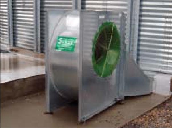
*Each bin is equipped with four 30hp Sukup centrifugal fans.*
