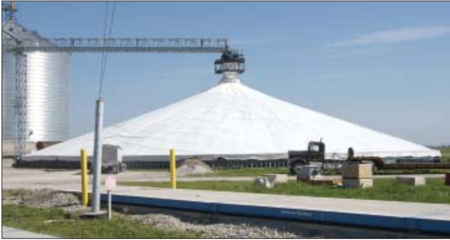
*Closeup of the smaller of two LeMar center fill temporary storage piles. This one is 250 feet in diameter and holds about 1 million bushels. Newest Weigh Tronix truck scale is in the foreground.*
