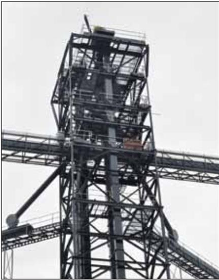
*Receiving legs feed into a five-hole Schlagel electronic triple distributor.*
