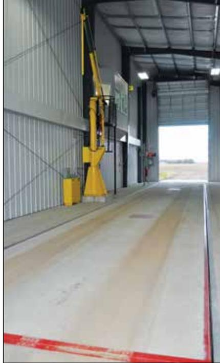
*Enclosed scalehouse adjacent to the facility office building includes an 80-foot Rice Lake truck scale, Gamet truck probe, and CompuWeigh SmartView screens.*
