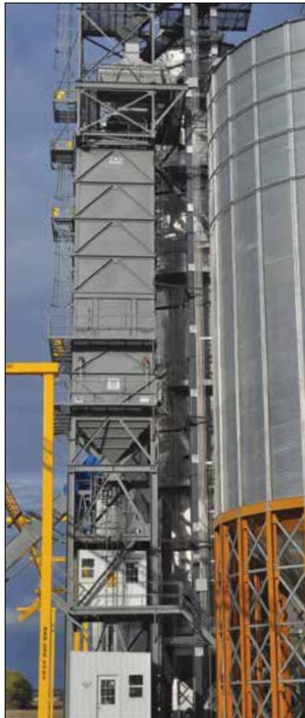
*The terminal's 80,000-bph bulk weigh loadout scale from C&A Scales is topped by an Intersystems gravity screener.*
