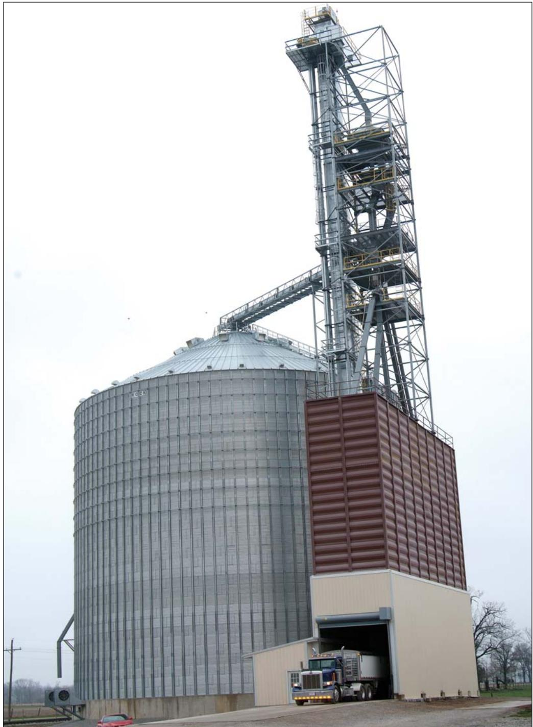
*New 735,000-bushel steel annex at the Harvest Land Cooperative elevator in Hagerstown, IN, including, from left, Brock grain storage tank, receiving and loadout shed with four 8,000-bushel plus one 1,500-bushel Baker Rullman square steel bins, and LeMar tower housing a 20,000-bph InterSystems leg, InterSystems gravity cleaner, and two Schlagel distributors. Photo by Ed Zdrojewski.*
