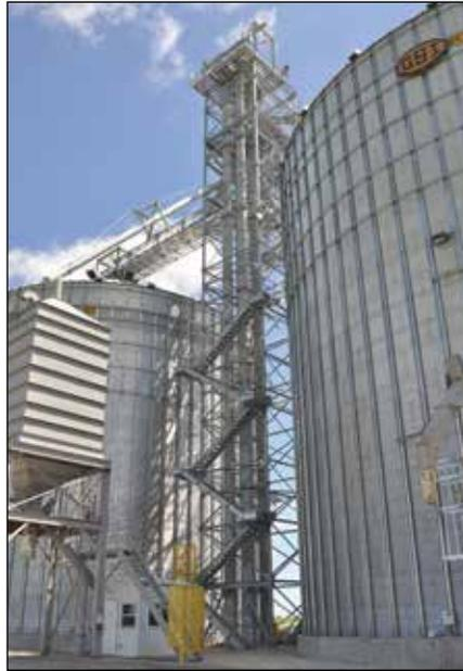
*Grain handling equipment includes a pair of 15,000-bph InterSystems receiving legs supported by a LeMar tower and a 2,500-bushel truck-loading surge tank.*
